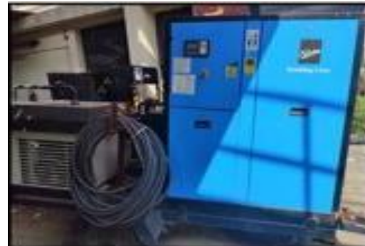
After – 4 Nos small portable compressors fixed where its is required.
